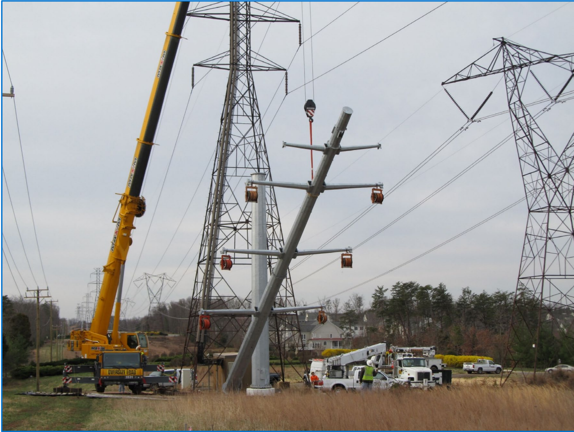
Cranes help assemble the pole pieces.
