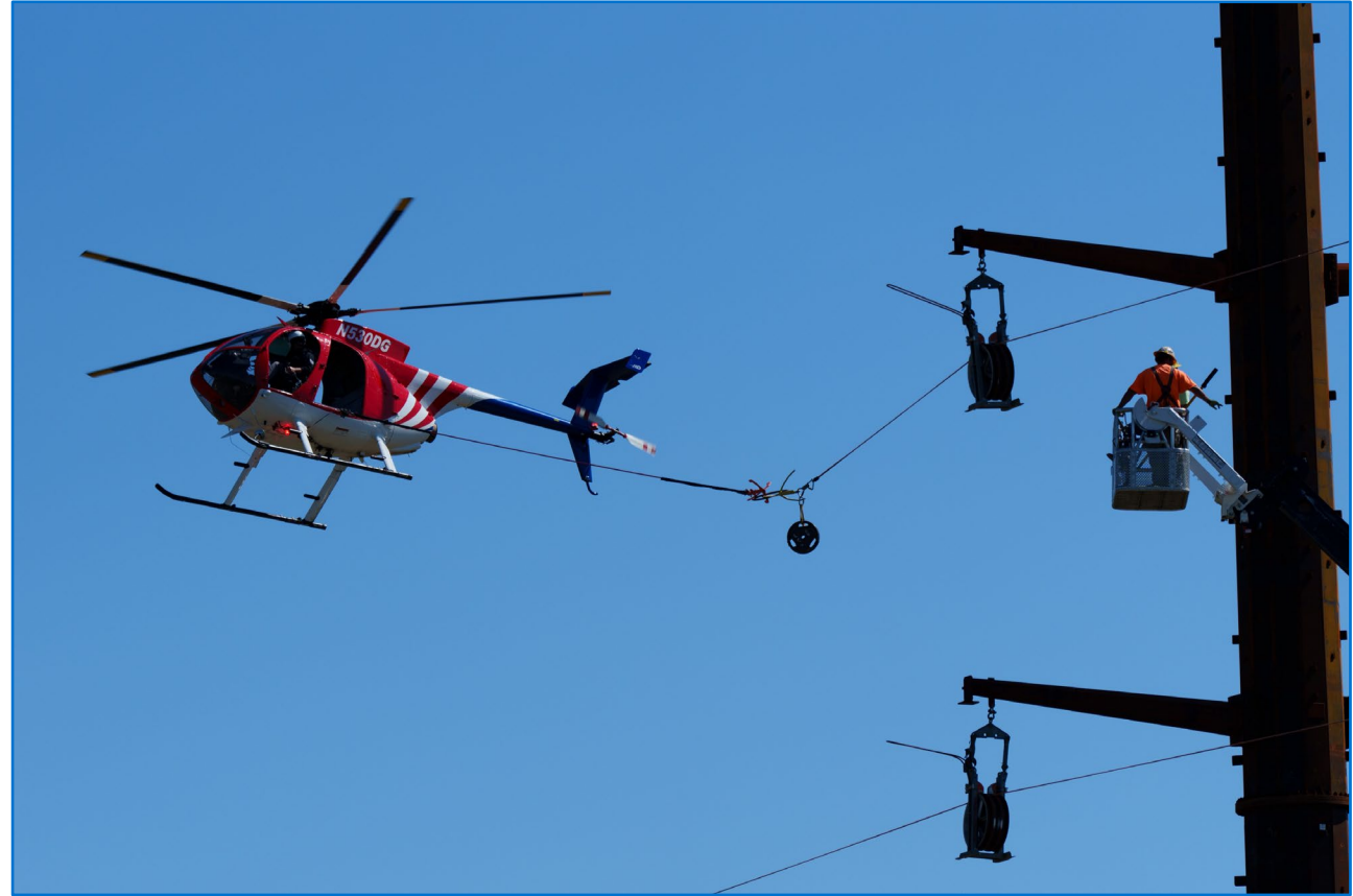
Helicopter helps install lines.
