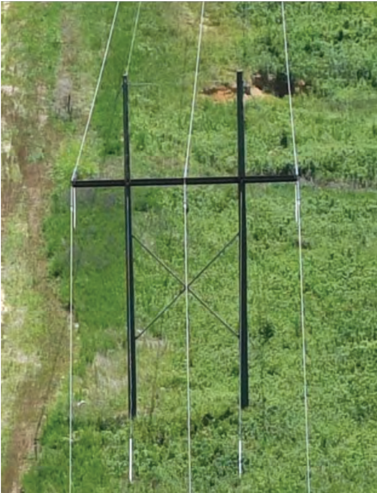
Existing Single Circuit Double Deadend H-frame
