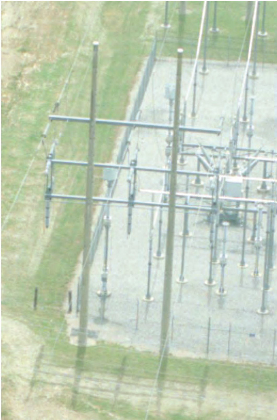
Existing Single 230 kV Circuit Switch
