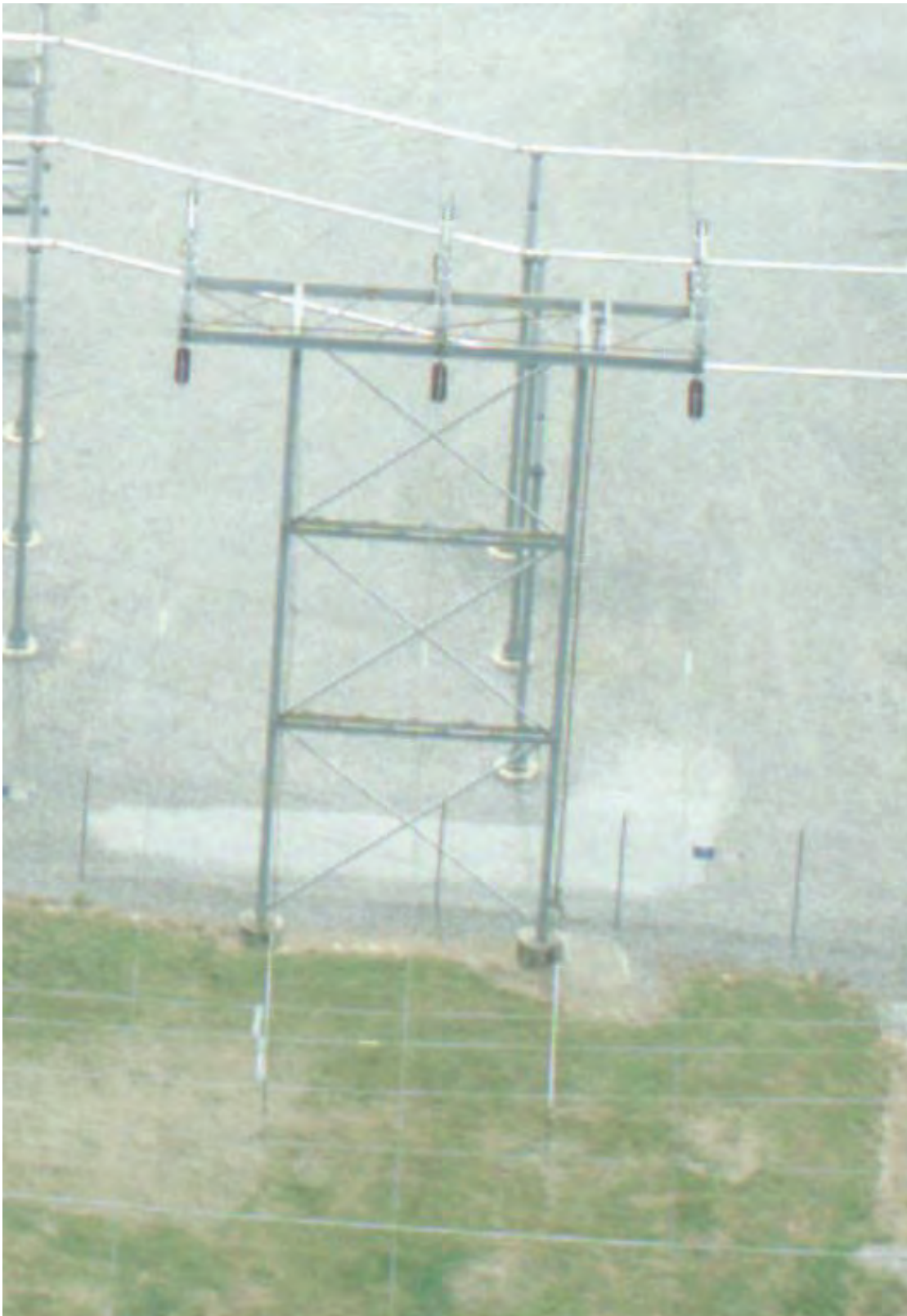
Existing Single 115 kV Switch Structure
