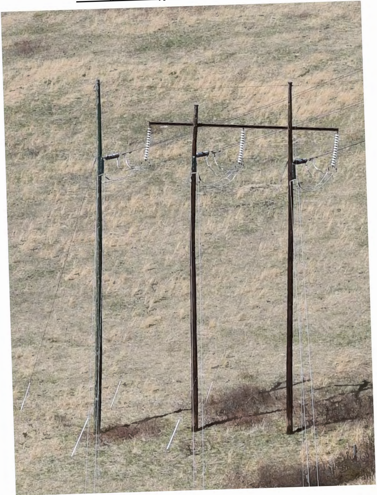
Existing Structure Type for Line #293: Wood Three-Pole
