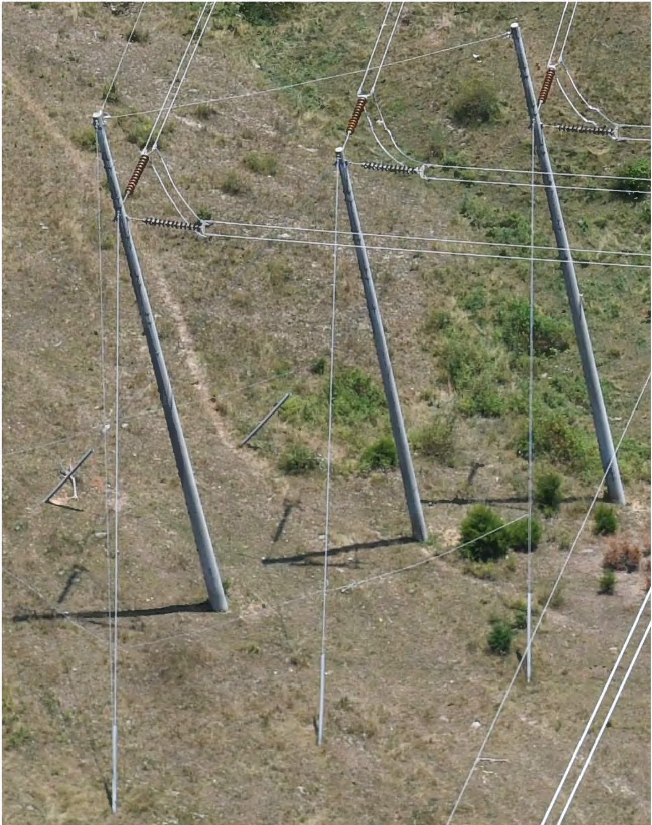
Existing Structure Type for Line #293: Concrete Three-Pole
