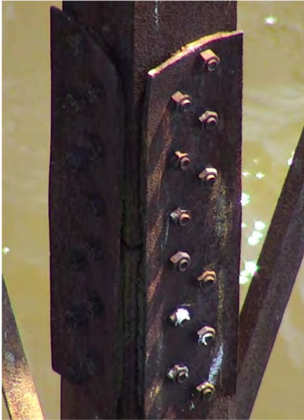
Severe Packout & Steel Damage
