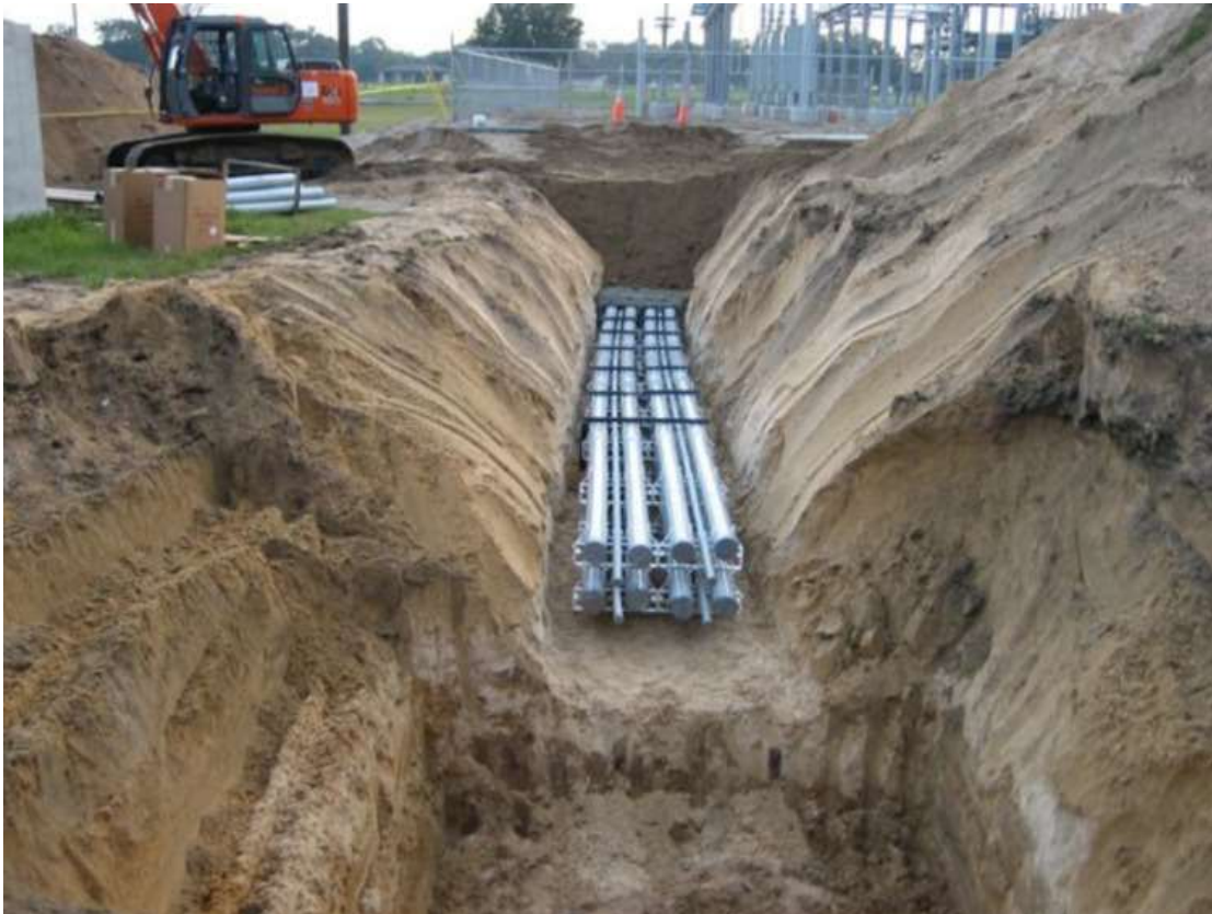
Figure 2-1: Duct Bank System Example
