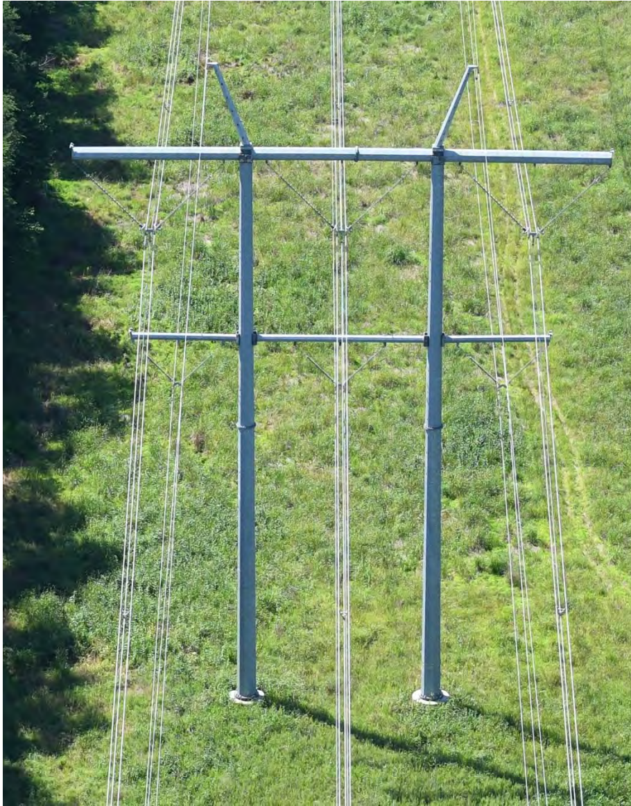
II.B.6.b.v – Double Circuit 500kV/230kV H-Frame Suspension Structure
