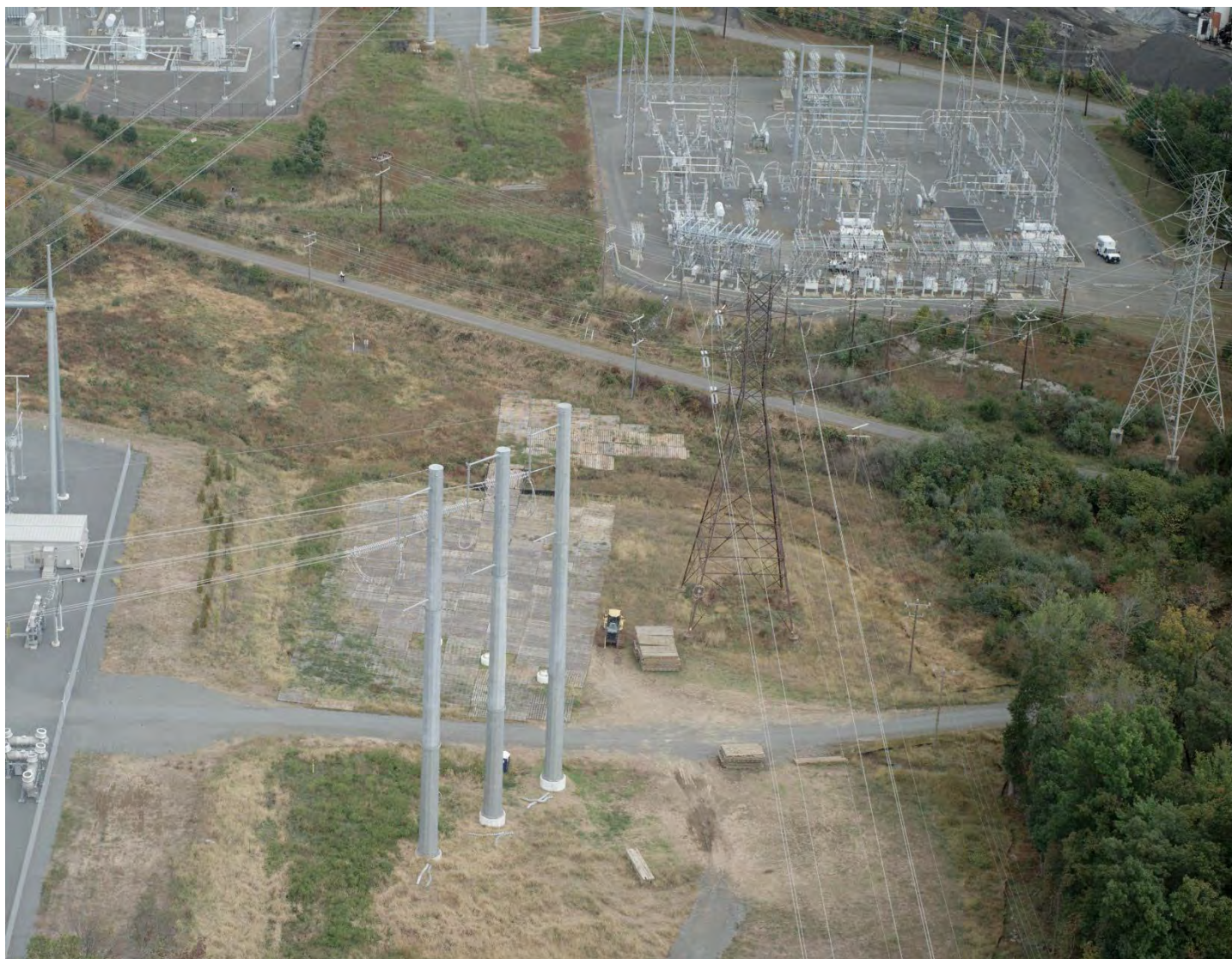
Str. 558/1856 Galvanized 3-Pole to be Removed
