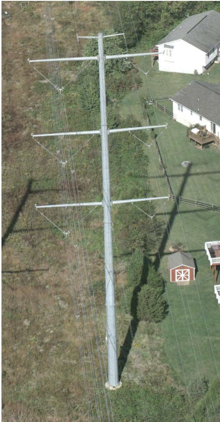
II.B.6.b.ii – Double Circuit 500 kV / 230 kV Suspension Structure
