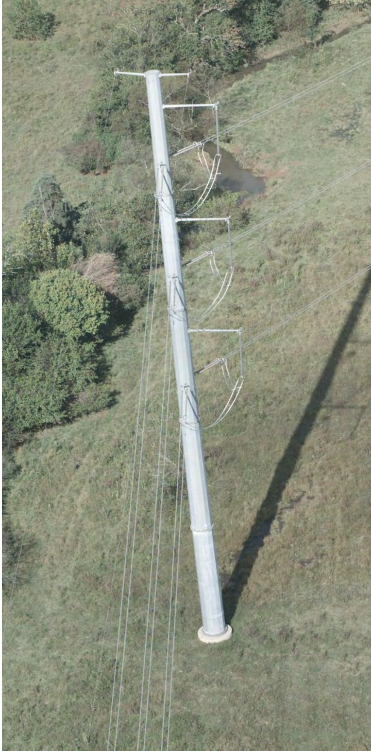
II.B.6.b.viii – Single Circuit 500kV 1-Pole Double Dead End Structure
