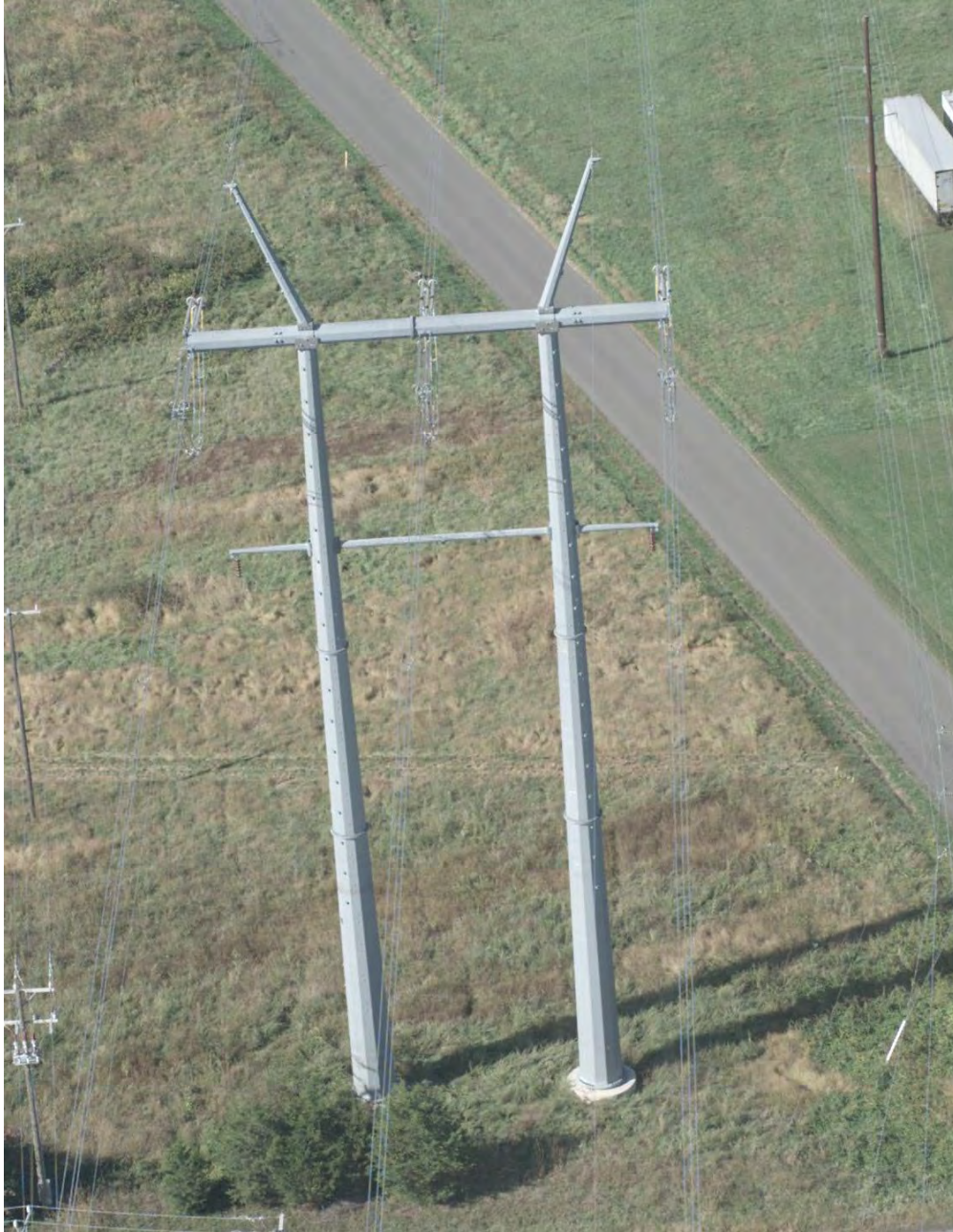
II.B.6.b.iv – Double Circuit 500kV/230kV H-Frame Double Dead End Structure
