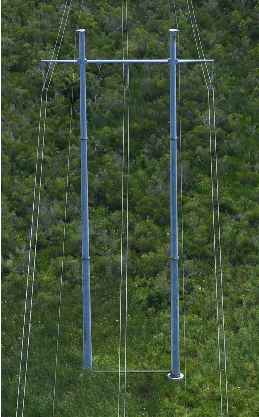
II.B.6.b.vii – Single Circuit 230kV H-Frame Structure
