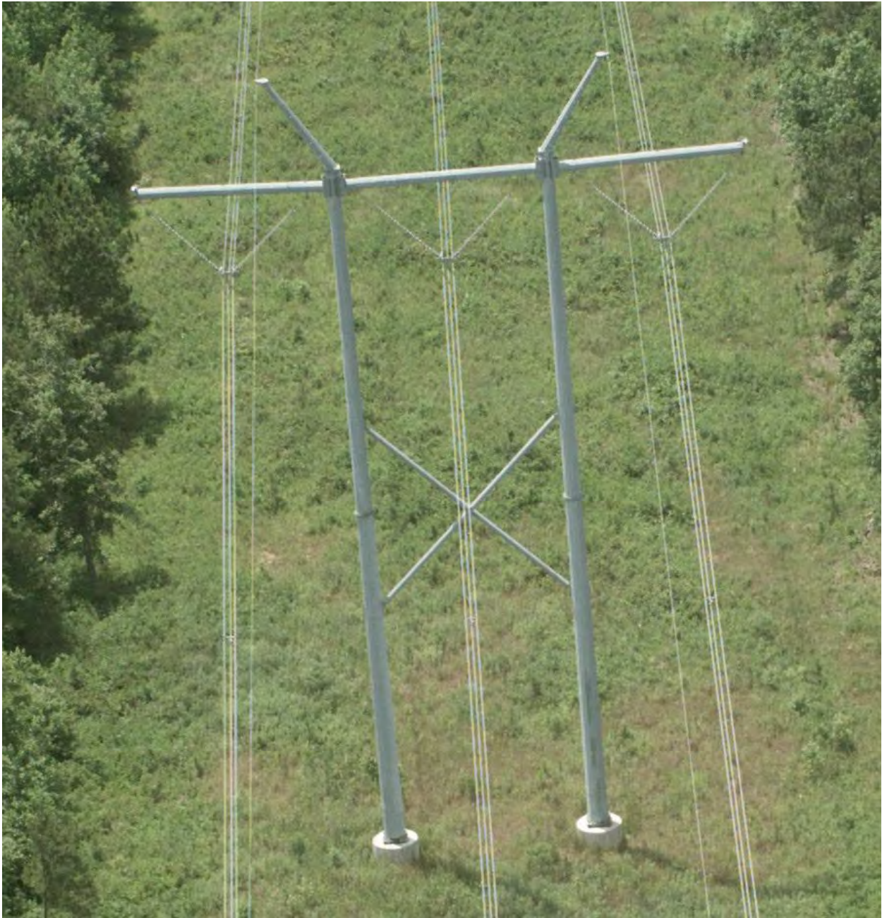
II.B.6.b.ix – Single Circuit 500kV H-Frame Structure
