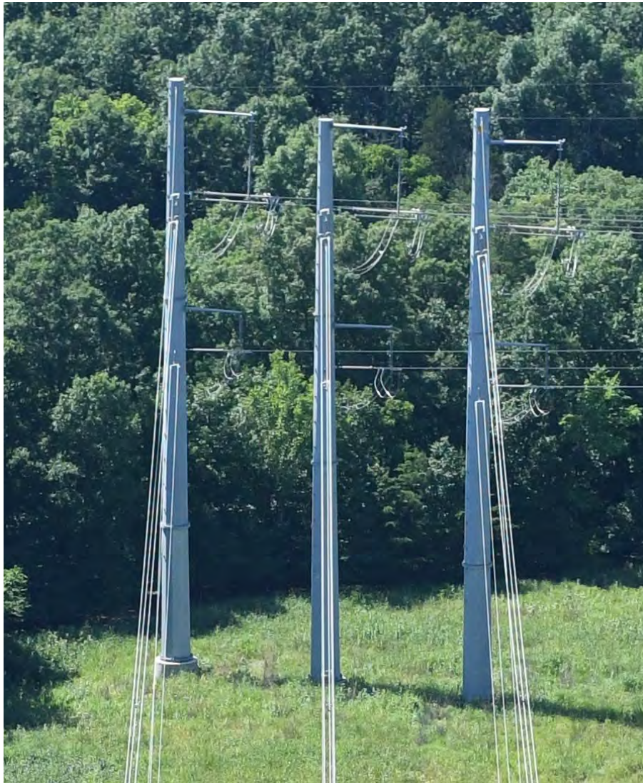
II.B.6.b.iii – Double Circuit 500kV/230kV 3-Pole Structure
