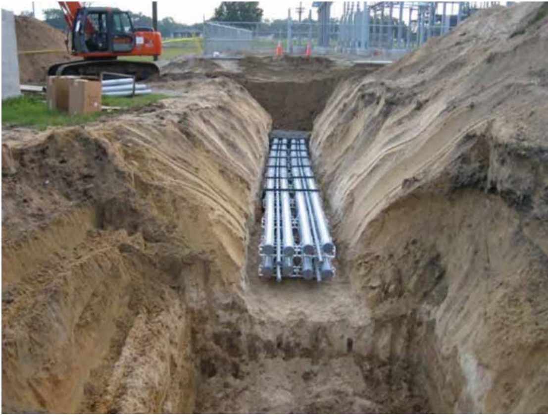
Figure 2-1: Duct Bank System Example
