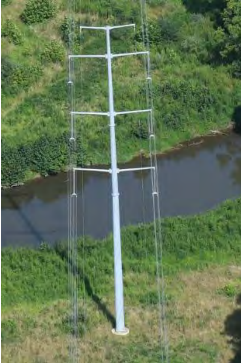
II.B.6.b.ii – Typical Double Circuit 230kV Monopole – Suspension
