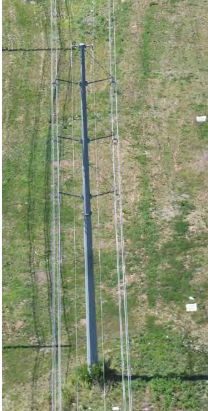
II.B.6.a.ii – Removal – Existing Strs. 2095/70 (2292/80) and 2095/71 (2292/81) along Route 606
