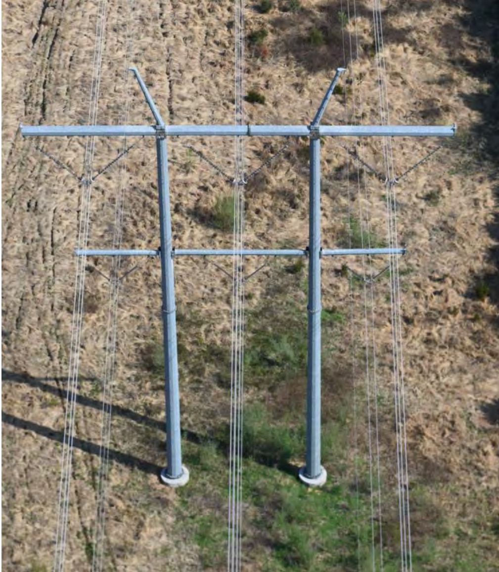
II.B.6.b.ix – Typical Double Circuit 500kV/230kV H-Frame – Suspension
