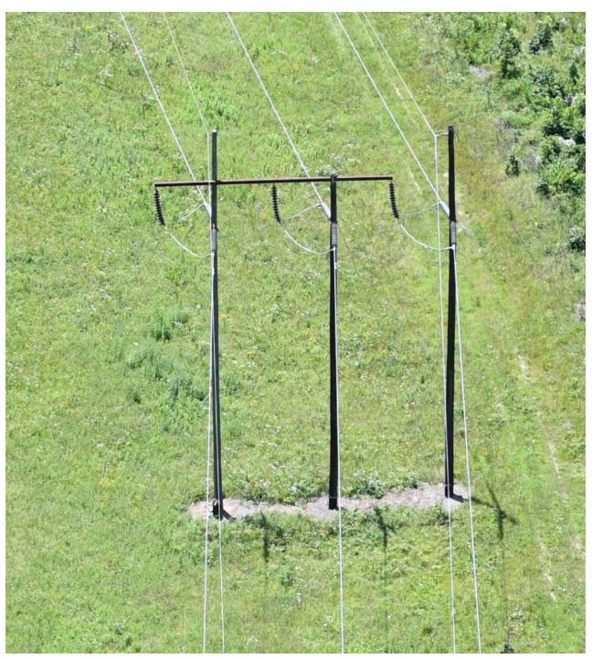
Existing Running Angle Structure Type For Lines #2201 and #254: Wooden 3-Pole
