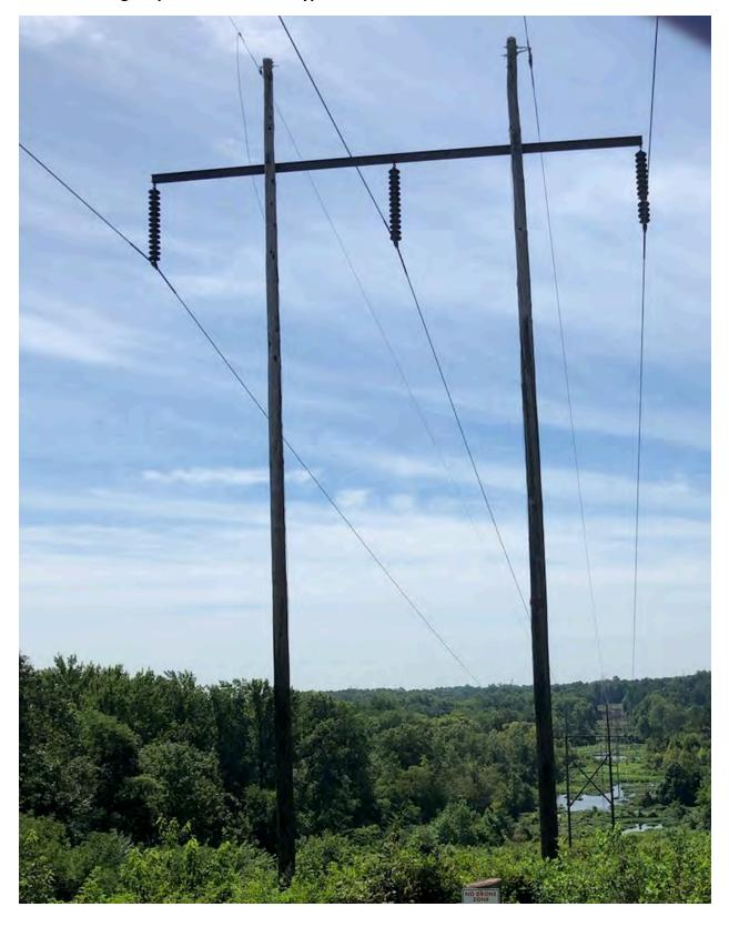
Existing Suspension Structure Type For Lines #2201 and #254: Wooden H-Frame
