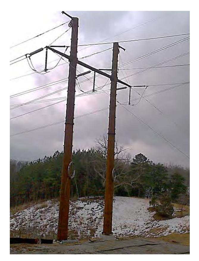
Proposed Double-Deadend Structure Type For Lines #2201 and #254: Weathering Steel H-Frame
