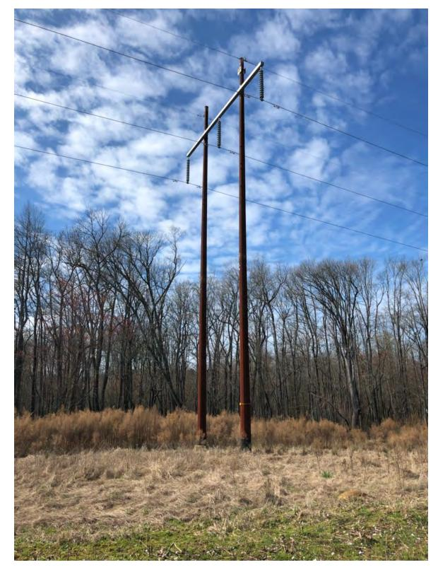
Proposed Suspension Structure Type For Lines #2201 and #254: Weathering Steel H-Frame
