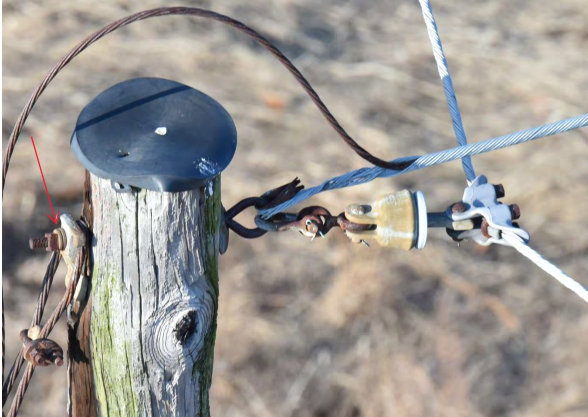
224/48, Preform thimble out of lay
