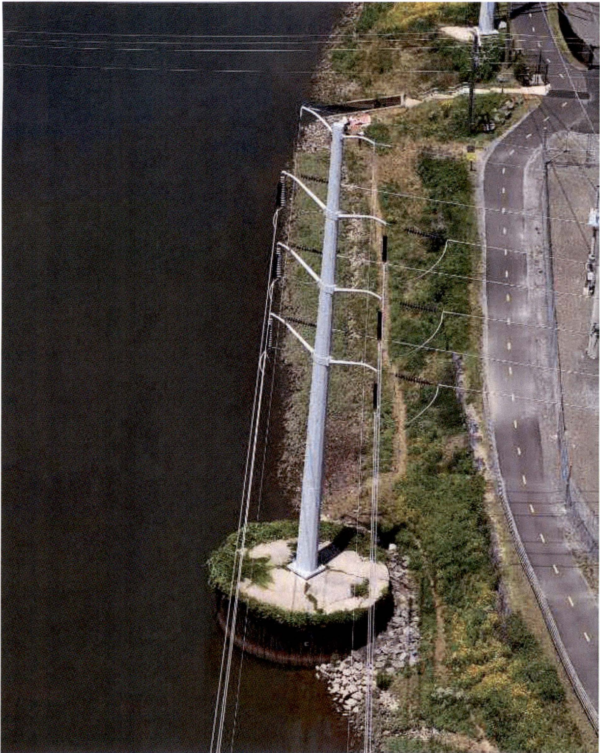
LOOKING WEST – EXISTING TRANSMISSION STRUCTURE #248/145 AND #2023/51 – 100' HIGH DOUBLE CIRCUIT STEEL POLE
