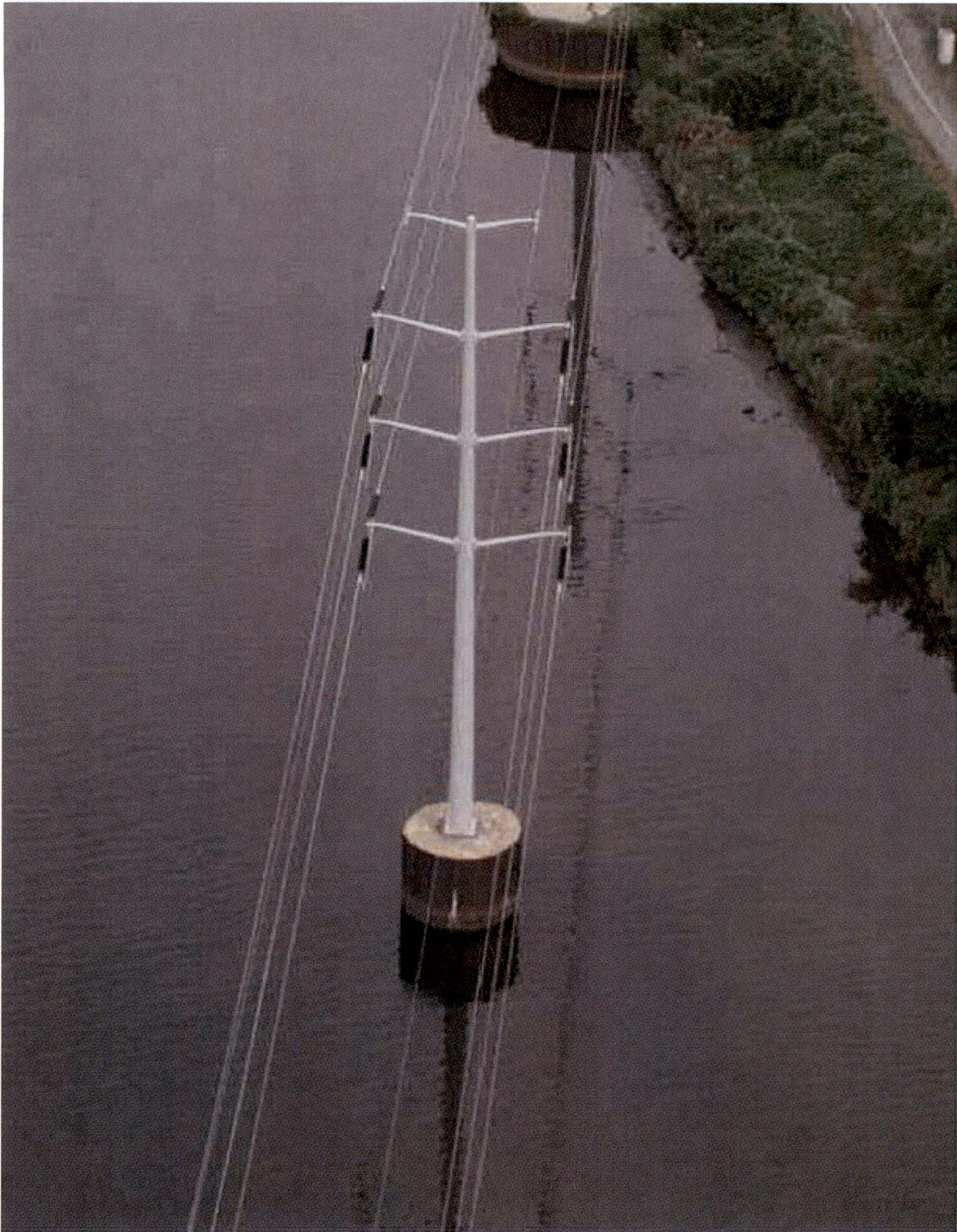
LOOKING NORTHWEST – EXISTING TRANSMISSION STRUCTURE #248/144 AND #2023/50 – 95' HIGH DOUBLE CIRCUIT STEEL POLE
