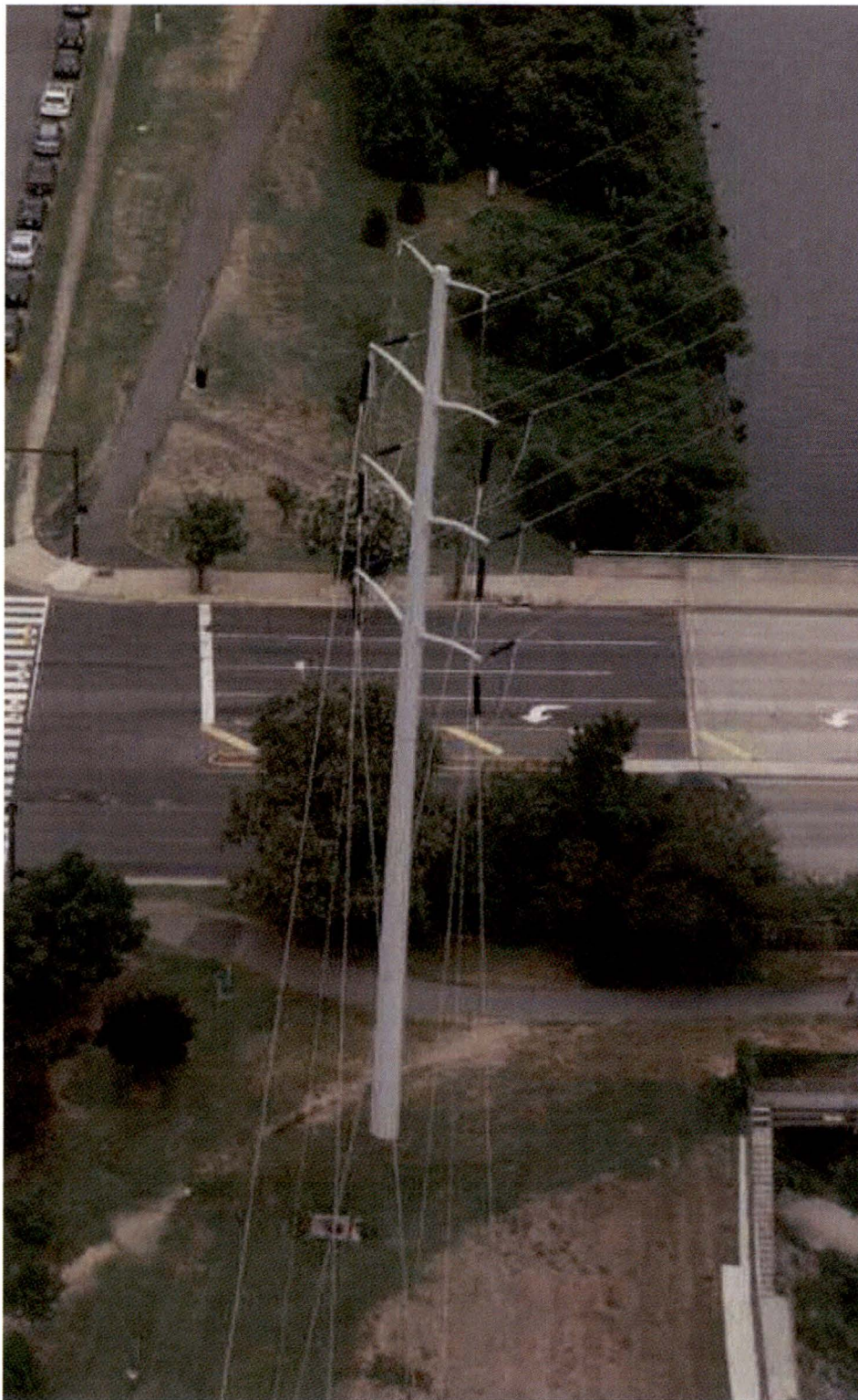
LOOKING NORTHWEST – EXISTING TRANSMISSION STRUCTURE #248/143 AND #2023/49 – 125' HIGH DOUBLE CIRCUIT STEEL POLE
