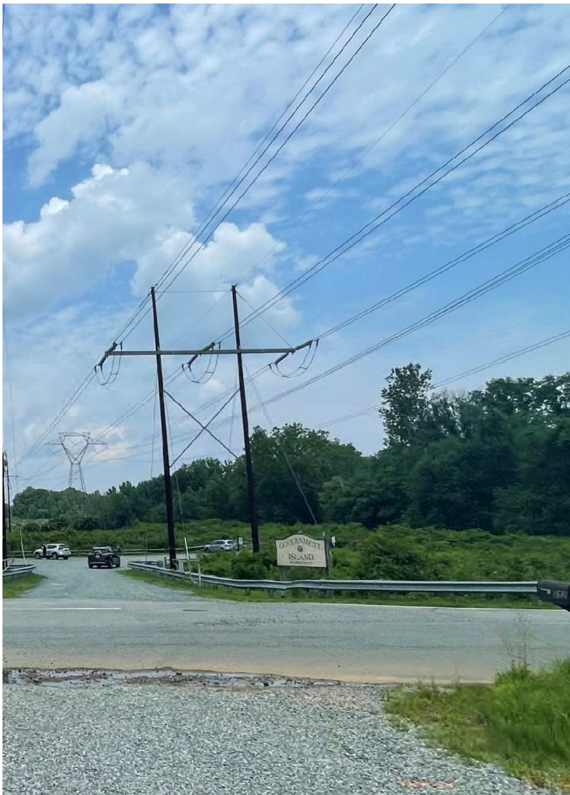
Existing Structure Type: 230kV Single Circuit Steel H-Frame (DDE)
