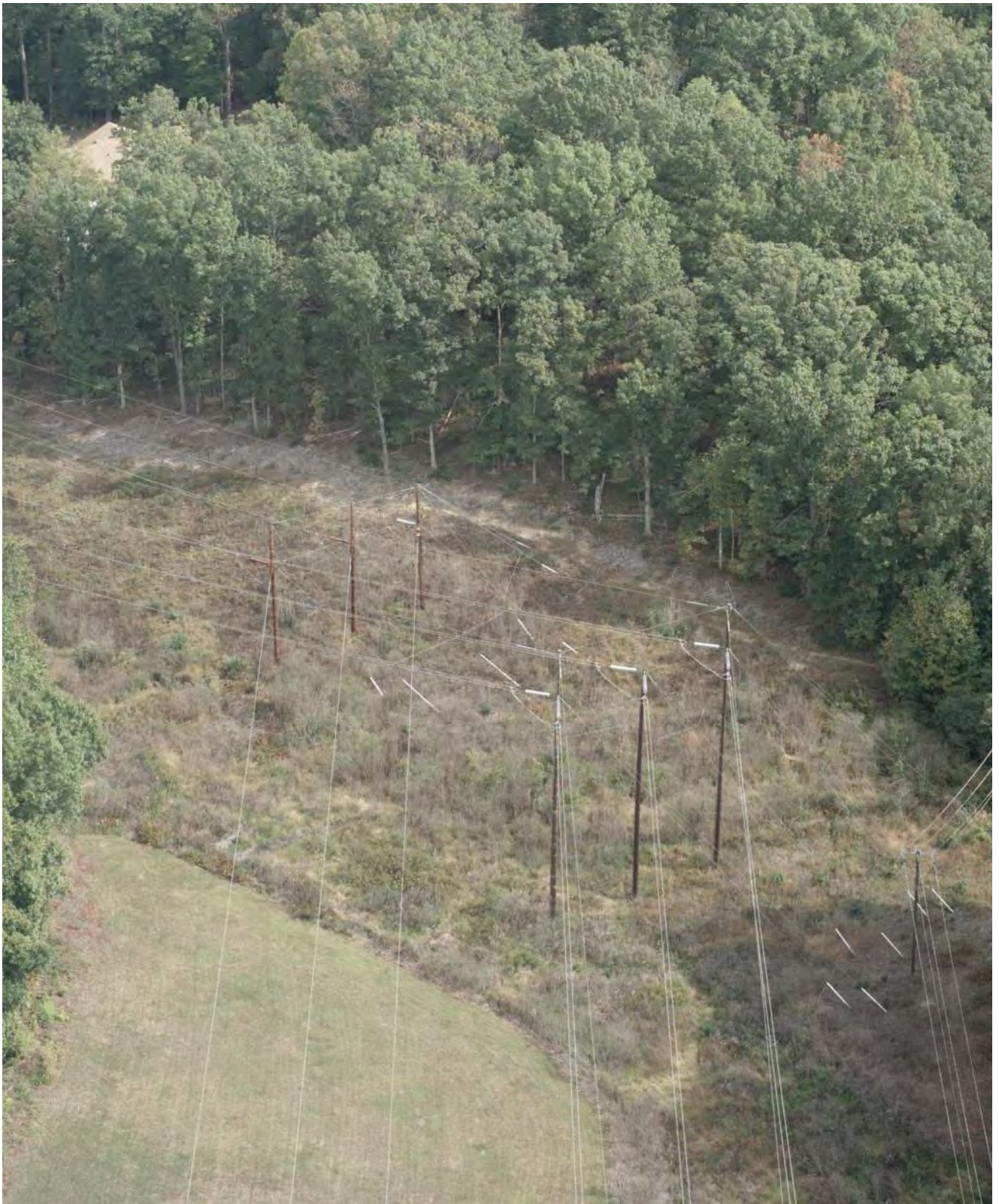
Existing Structure Type: 115kV (Left) And 230kV (Right) Single Circuit Wood 3-Pole (DDE)
