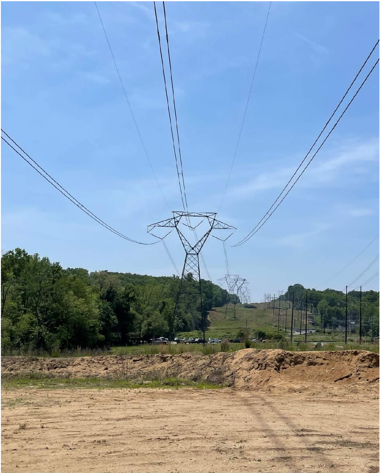
Existing Structure Type: 500kV Single Circuit Steel Tower (Tangent)
