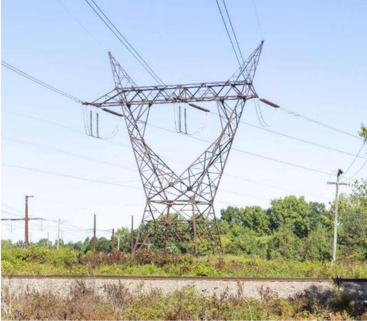
Attachment II.B.6.a.iii – Existing Typical SC 500kV Tower - Double Deadend (Weathering Steel)
