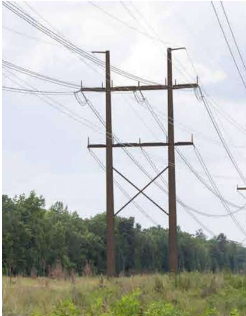
Attachment II.B.6.b.ii – Proposed Typical DC 500kV/230kV Engineered H-Frame – Double Deadend (Weathering Steel)
