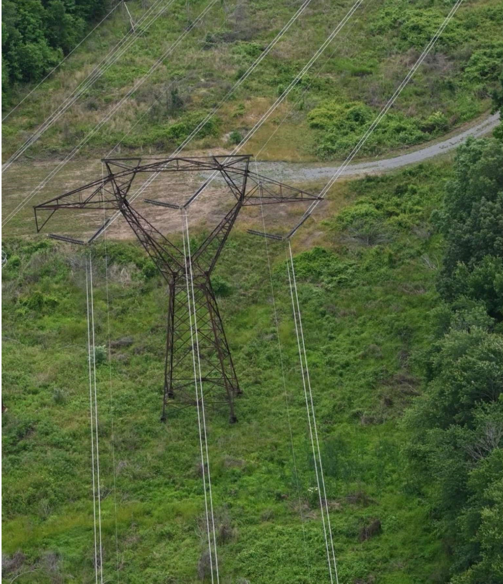
Attachment II.B.6.a.ii – Existing Typical SC 500kV Tower – Running Angle (Weathering Steel)
