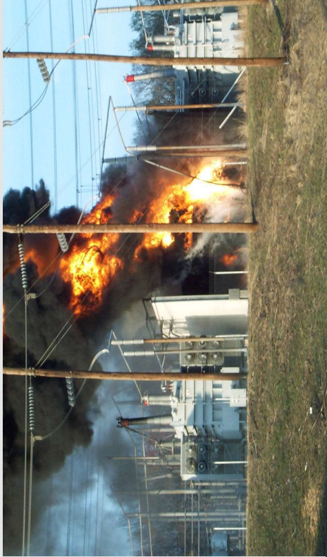
500 kV Transformer Failure in 2000
