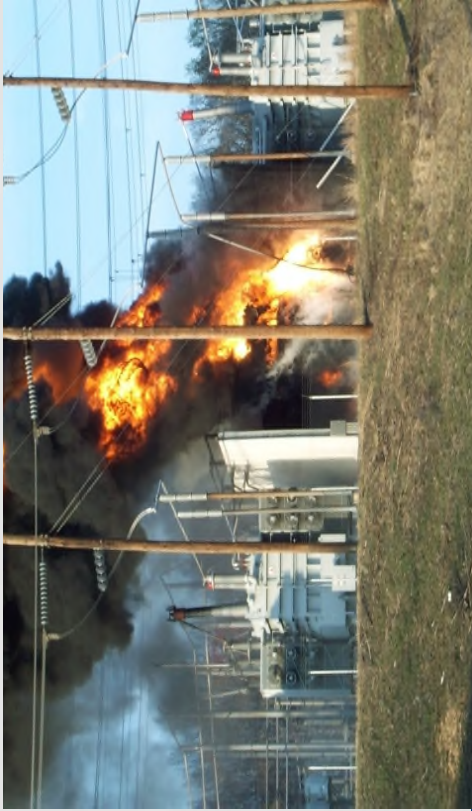
500 kV Transformer Failure in 2000
