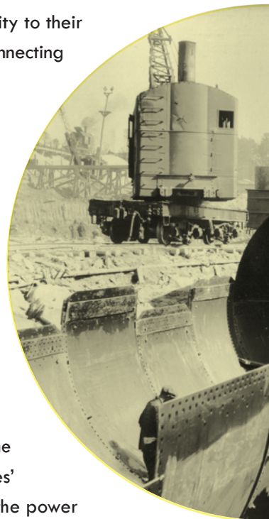
Figure 3. Construction of the penstocks
