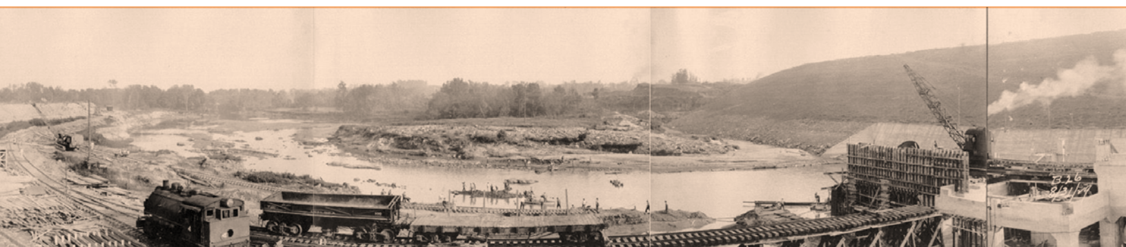
Figure 2. Railroads used in construction of the dam
